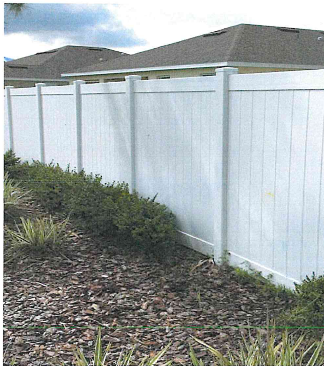
Figure 021: PVC privacy fencing at Del Tierra.
