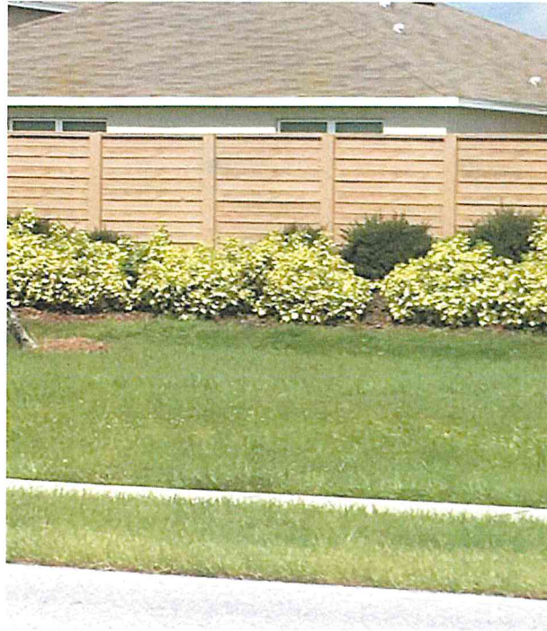
Figure 022: Rough sawn wood privacy fencing at Del Tierra.
