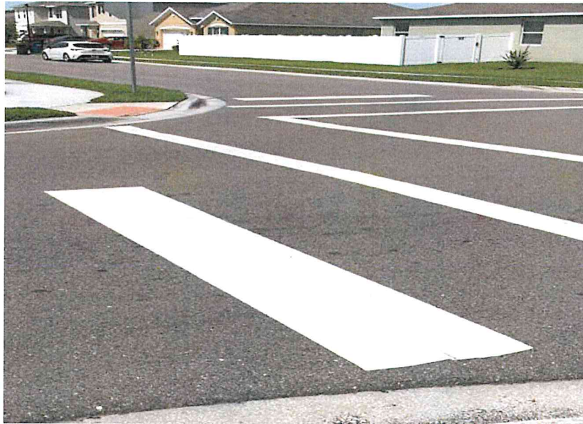
Figure 015: typical intersection and roadway pavement at Del Tierra.
