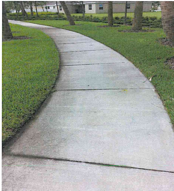
Figure 014: Typical 5 foot wide sidewalk at Del Tierra.
