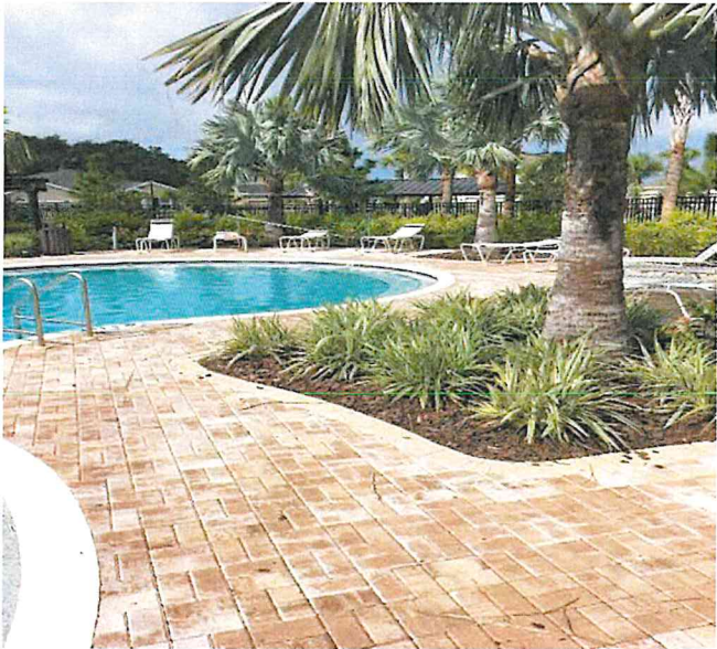
Figure 017: Pool and pool deck are in excellent condition.
